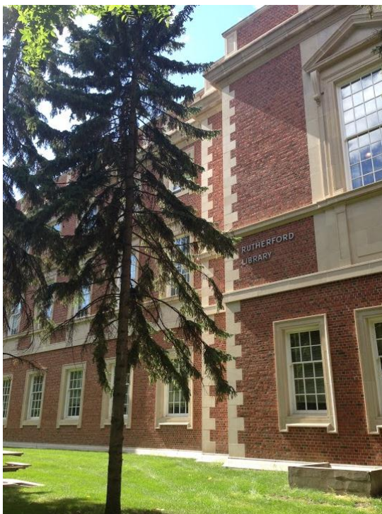
Rutherford Library (図書館外観)
