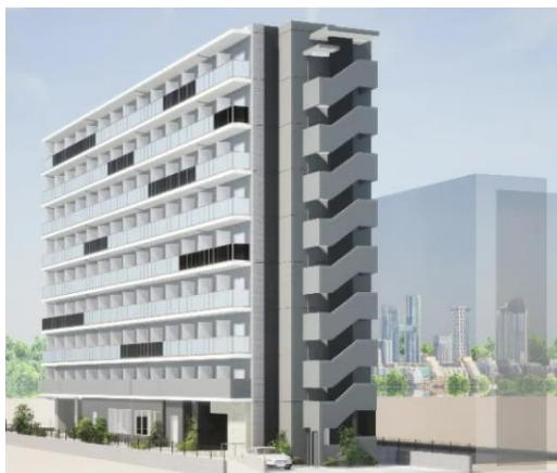
Exterior of the building / 外観
