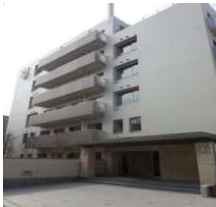
Exterior of the building / 外観
