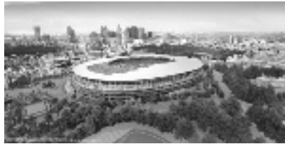
Figure 4: The new National Stadium design proposed by Kuma Kengo (image provided by the JSC)
