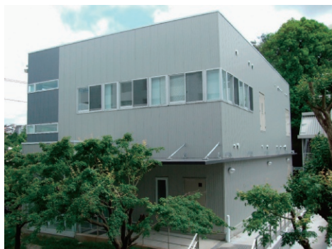
建物外観 External view of building
