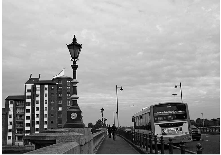
図2 Albert Bridge in Belfast
