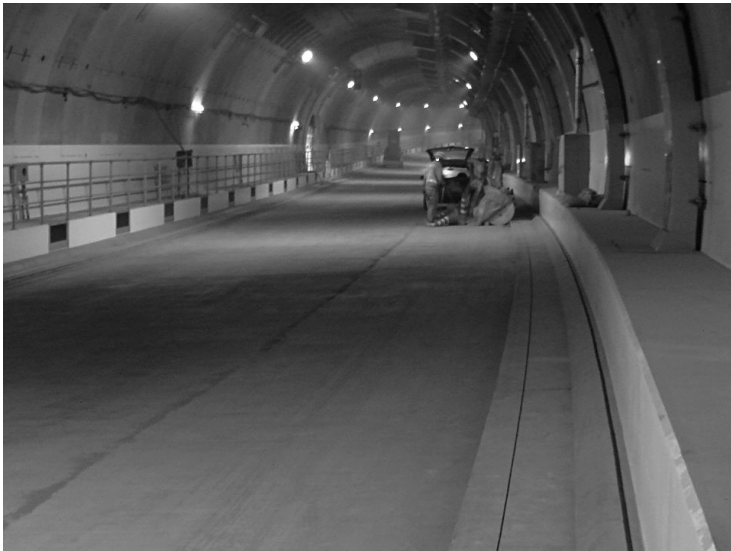
Figure 3. Ring Road 6 (Yamate Dori) was constructed in the form of a tunnel.
