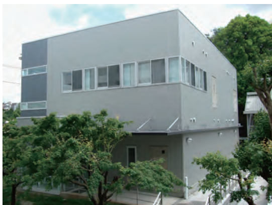
建物外観 External view of building
